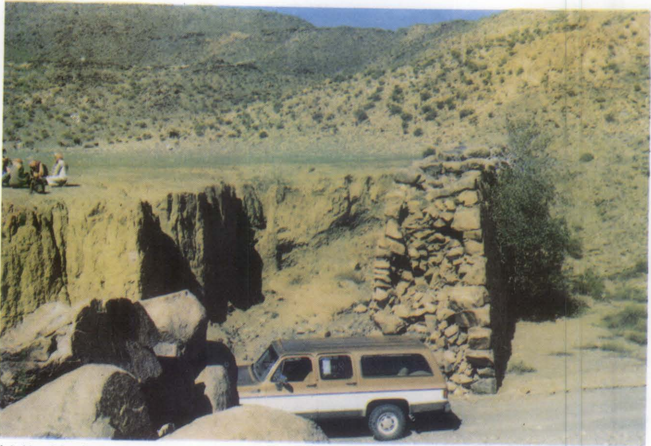
A. Sadd as-Salamah; silt and sediment have levelled the dam.
