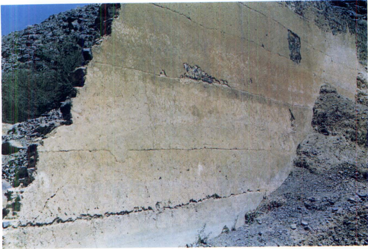
A. Sadd Thalbah; plaster on upstream face.
