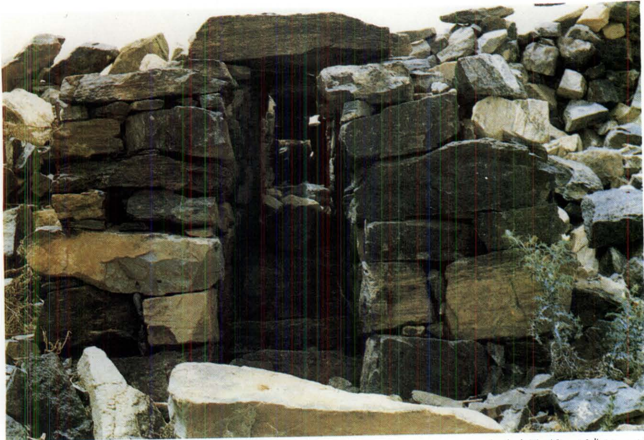
A. Sadd al-'Aqrab; water conduit in the middle.
