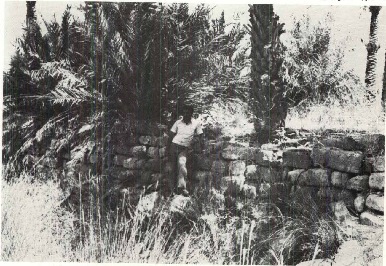
B. Embankment wall on south side of stream bed
